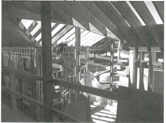
Framing at reconfigured entry
