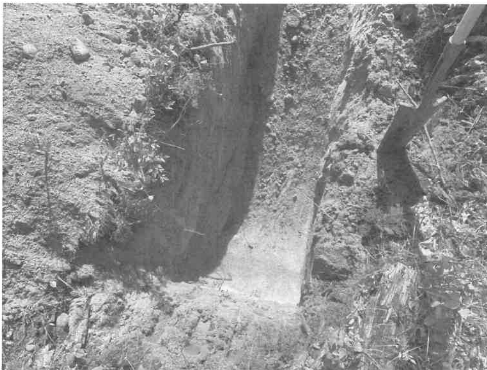
Photograph No. 14: View of Test Pit 17 showing Udipsamments soil with a wet substratum.
