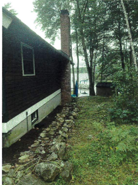
Photo #4 Existing House - Southeast View
