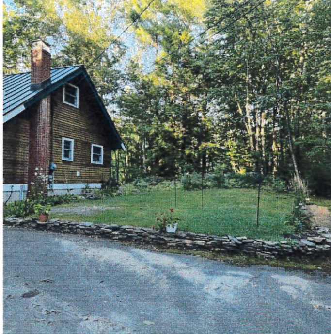
Photo #3 Existing House - Southwest View
