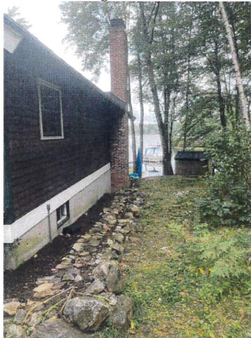
Photo #4 Existing House - Southeast View
