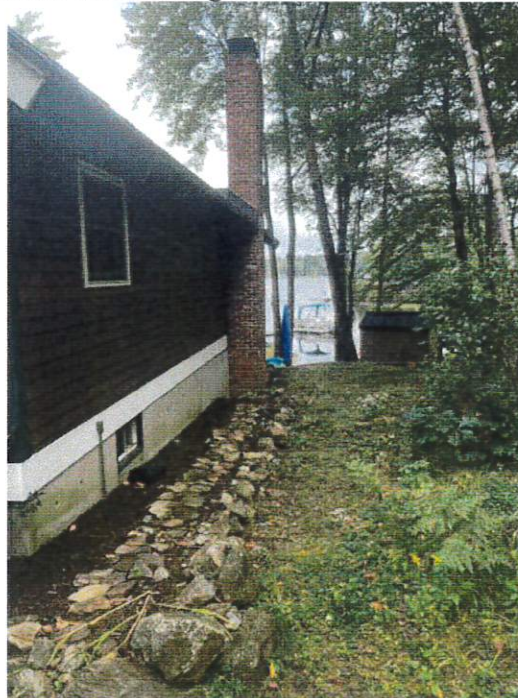
Photo #4 Existing House - Southeast View
