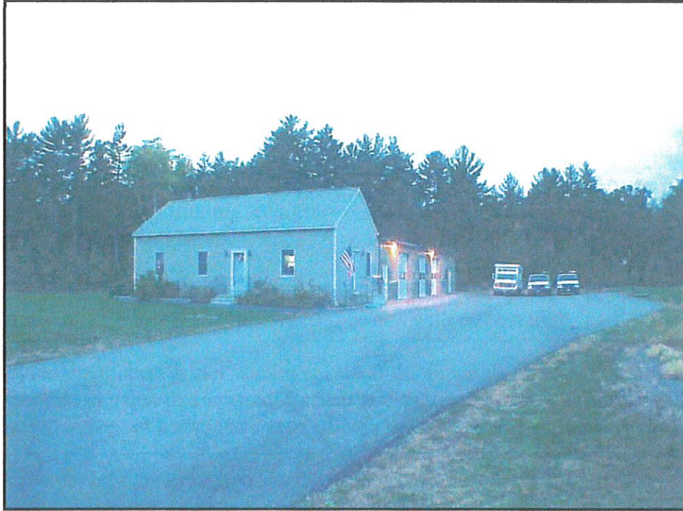
View of the subject property from Commerce Way.
