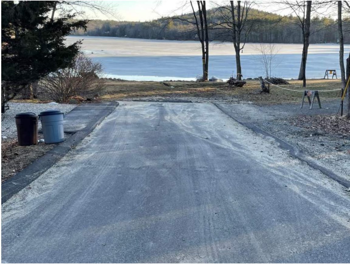
Figure 5 Looking South. Width is 15'-0" with 2' shoulders.
