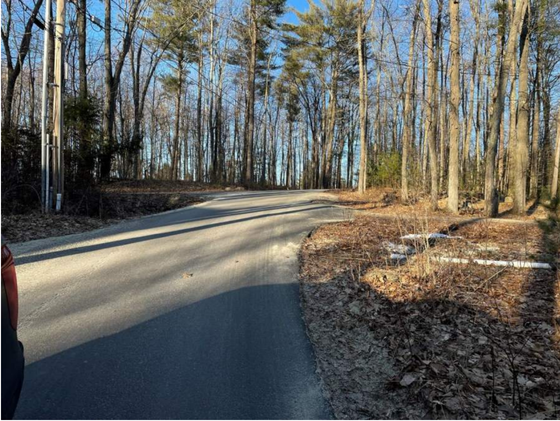
Figure 7 Looking north Width is 15'-0" with 2' shoulders.
