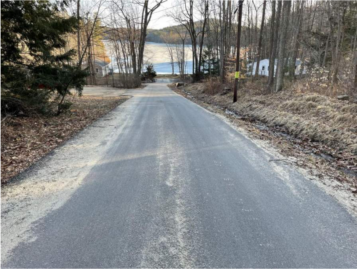
Figure 8 Looking south Width is 15'-0" with 2' shoulders.
