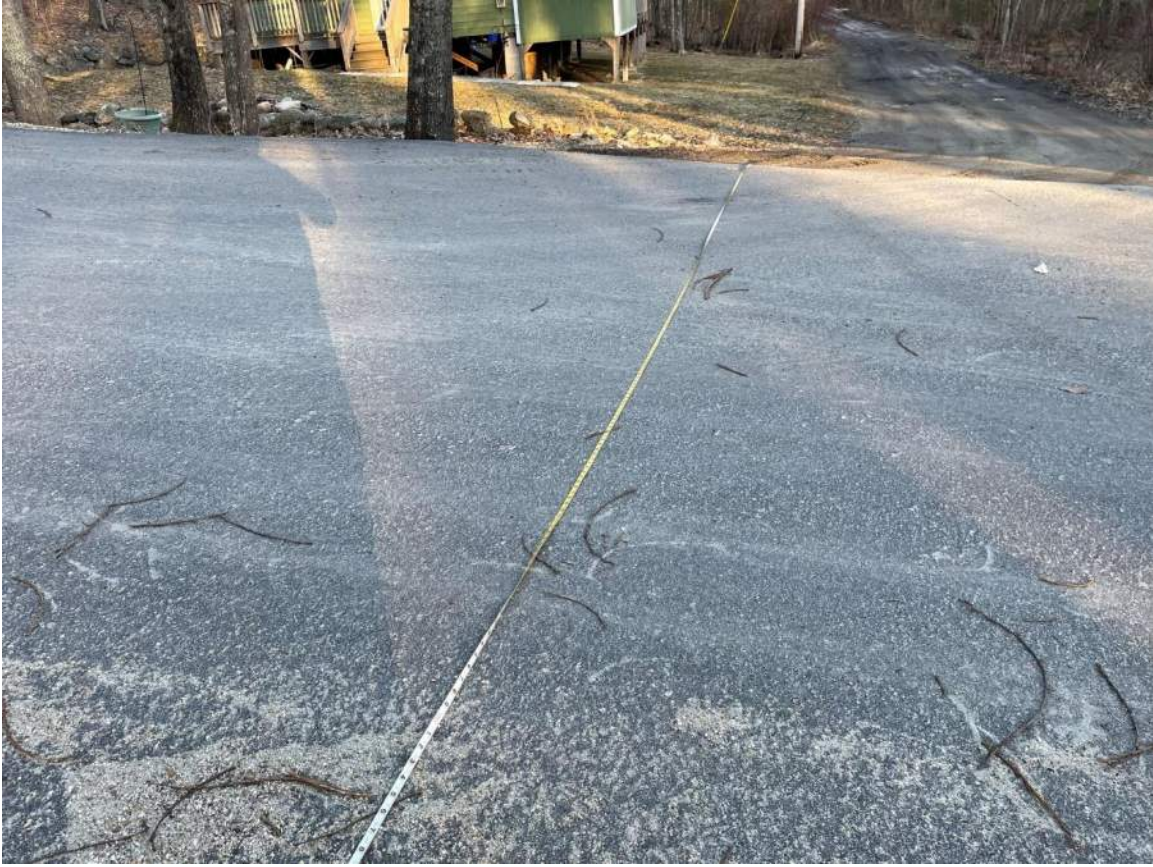
Figure 2 at intersection of Golf Course way and Eagle Drive. Width is approximately 21' with 2' shoulders.
