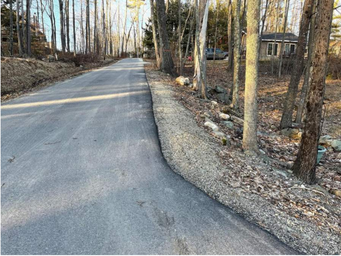
Figure 4 Looking North. Width is 15'-0" with 2' shoulders.
