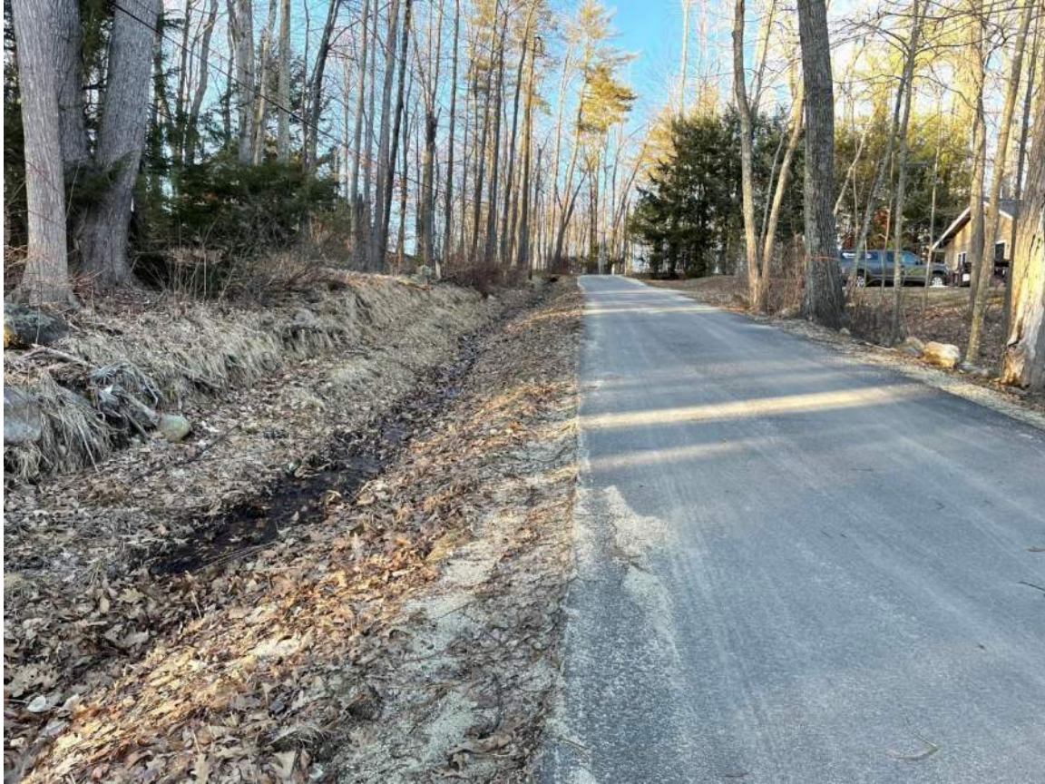
Figure 3 Looking uphill. Width is 15'-0" with 2' shoulders.
