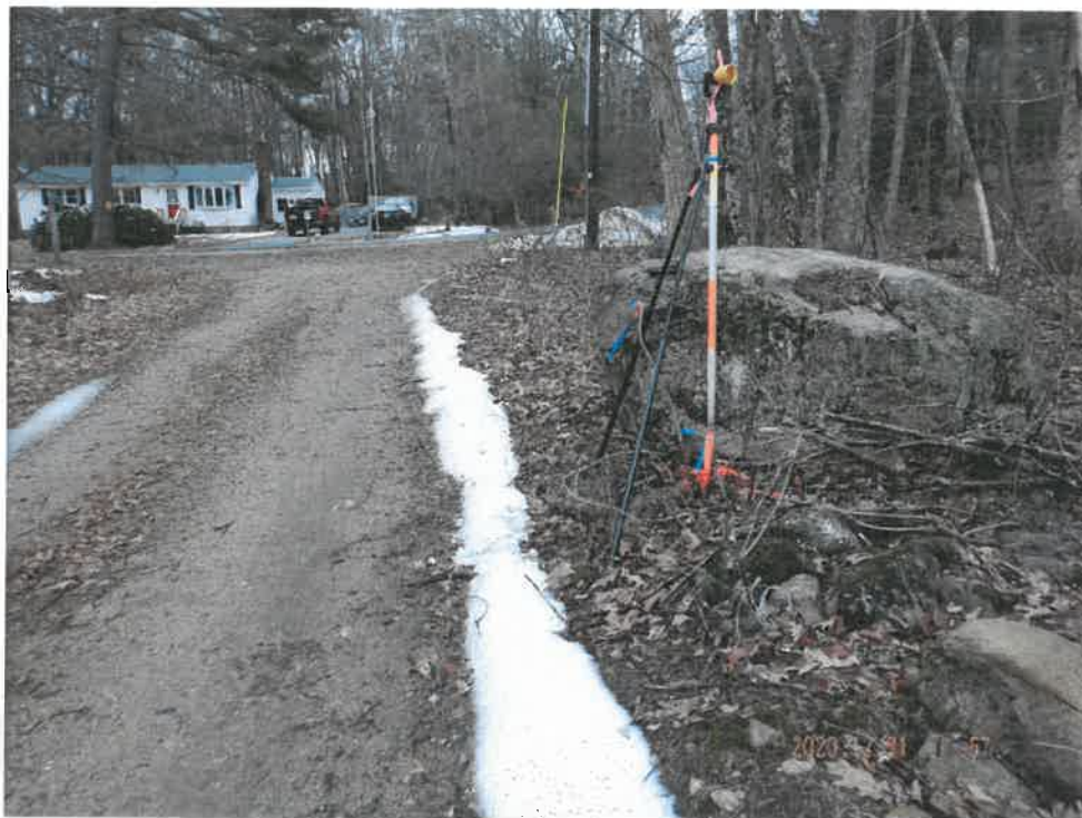
LOOKING EAST FROM EXISTING GRAVEL DRIVEWAY
