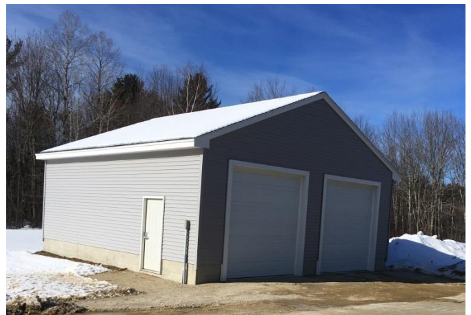
Fire and Rescue Department Storage Shed [Photo Credit: Rick Walker]
