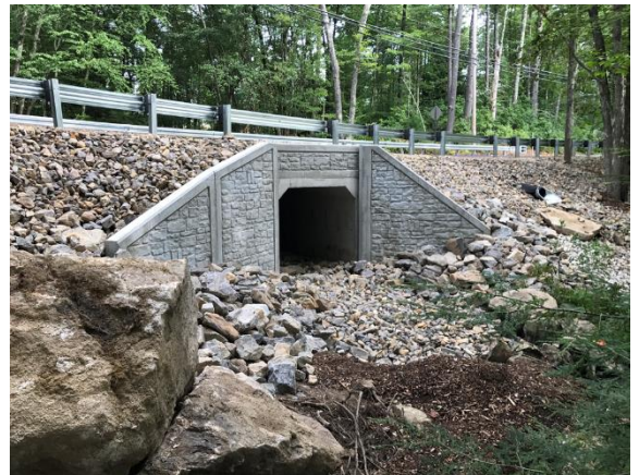
Young Rd. Culvert Replacement [Photo Credit: Marcia Gasses]
