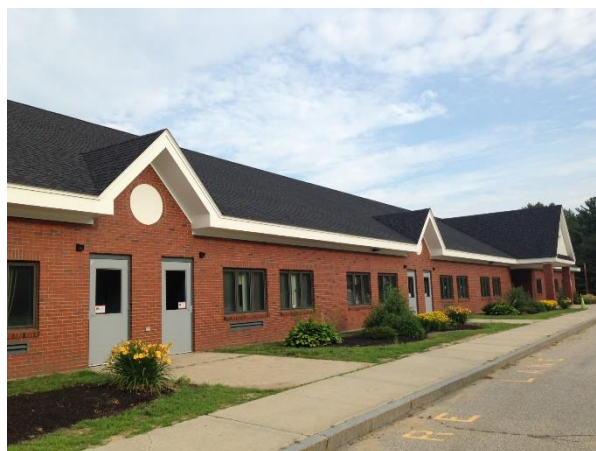
Barrington Elementary School [Photo Credit: SAU 74]
