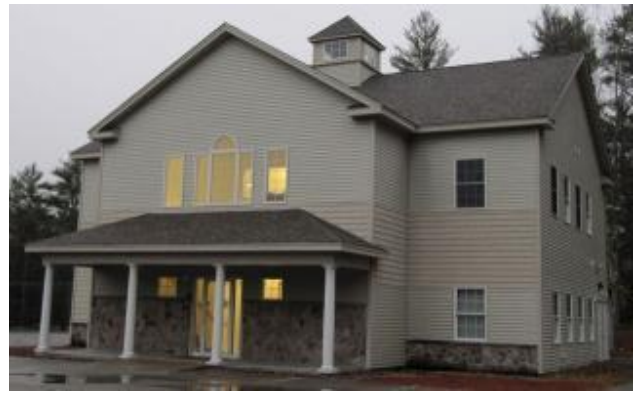
Existing Town Hall [Photo Credit: Town of Barrington]
