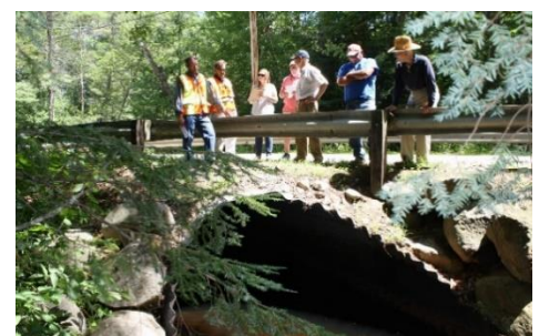
Mallego Road Crossing [Photo Credit: NHDOT]
