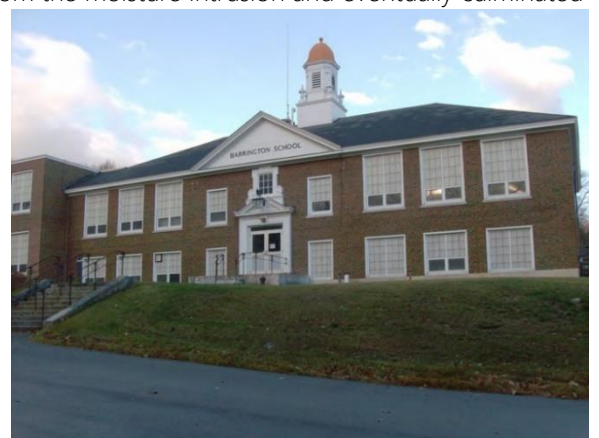
Former Town Hall [Photo Credit: H.L. Turner Group Inc.]
