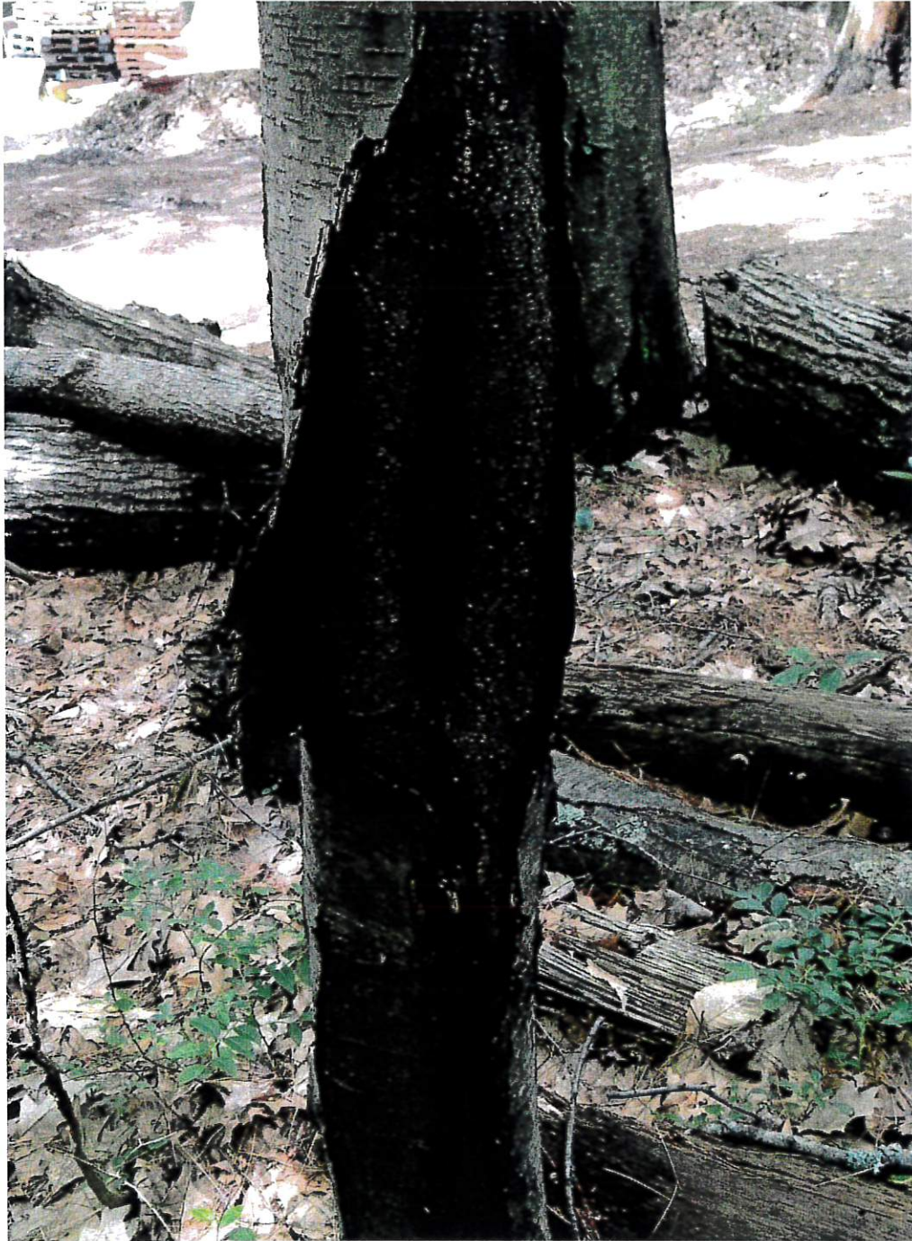
Figure 2. This tree shows an example of a tree that has a large trunk wound. Most likely the result of being hit by a fallen tree. A large pocket of decay is visible and this tree will be an unacceptable risk to failure as it gets larger.
