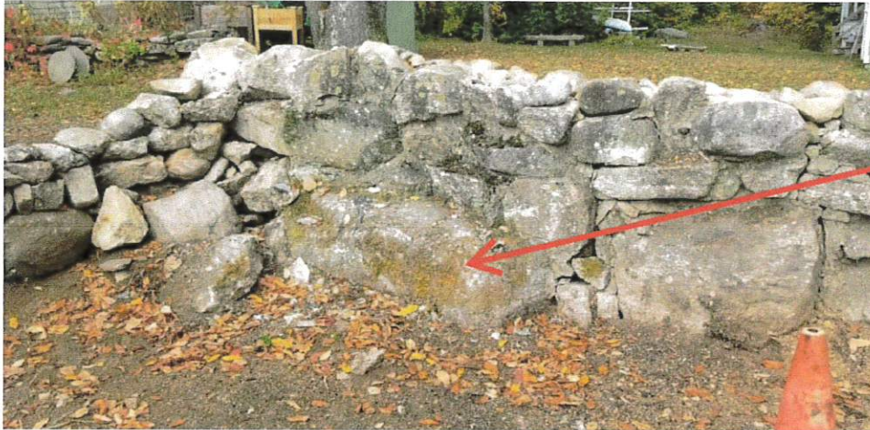
Old Foundation built over ledge
