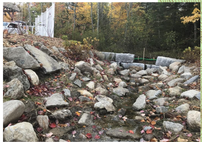
Restored inlet with natural Granite stone Weir
