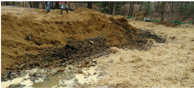
Wetlands violation restoration monitoring
