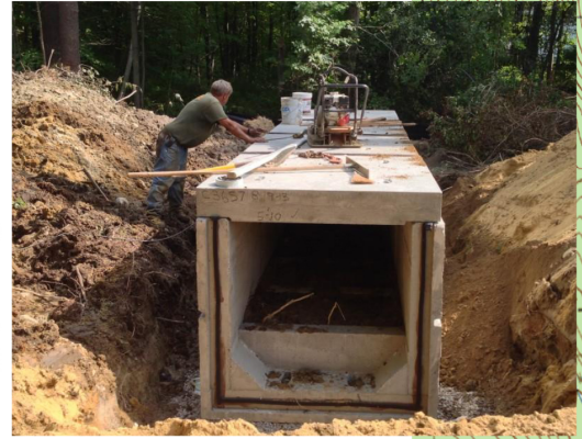
“Bottomless” Box Culvert
