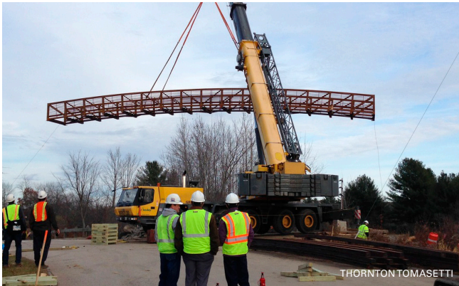
River Point Pedestrian Bridge, Falmouth, ME
