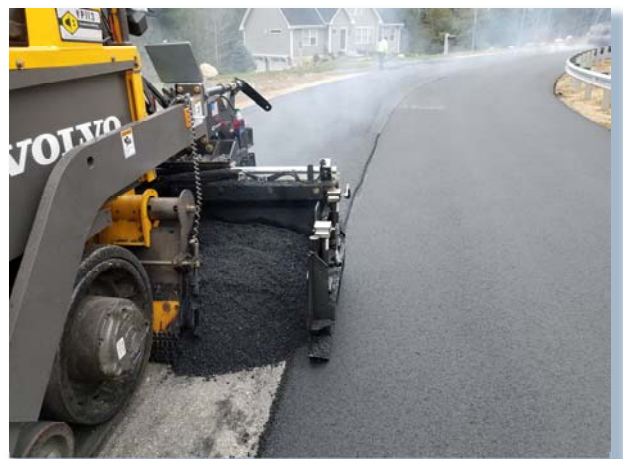
Wearing course pavement joint overlap
