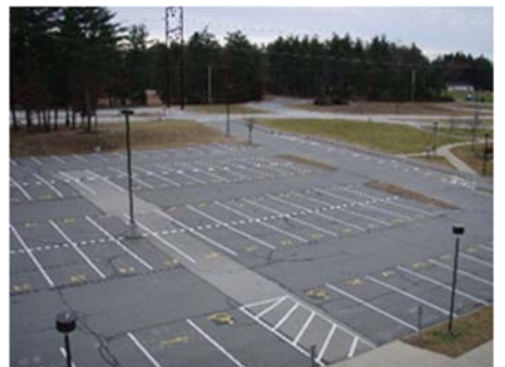
Campus evaluation, including pavement surface
