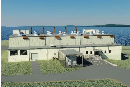
Naval Power Plant, Cutler, ME
