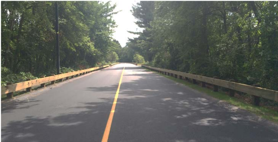
Reconstruction of Entrance Roads
