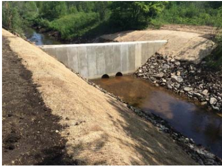
Tacan drainage weir
