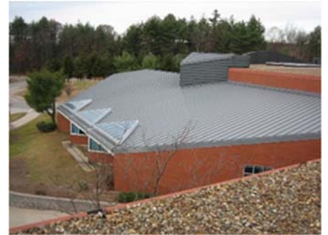
New aluminum roof system
