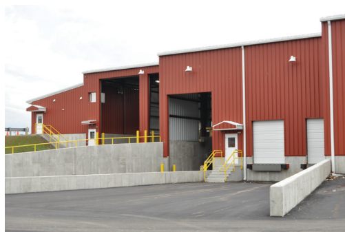
Public Work Facilities
