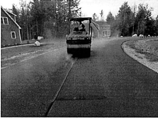
Figure 5 – Compaction of joint
