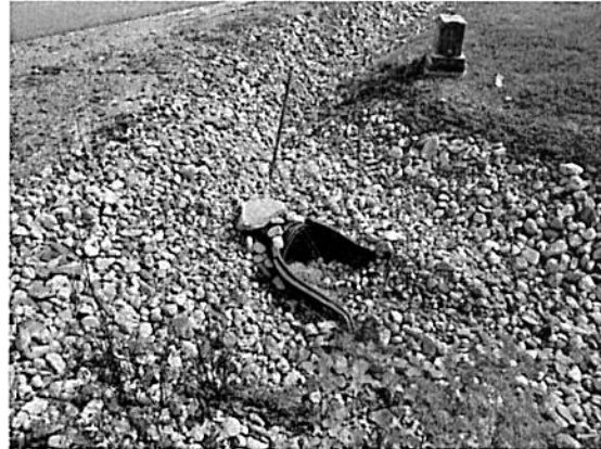
Figure 2 – Stabilize all flared-end sections
