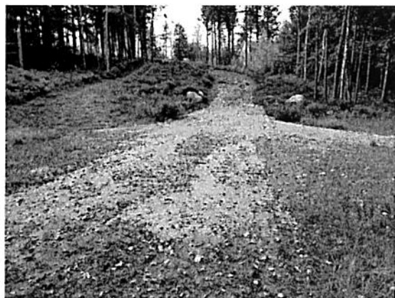
Figure 4 – Stabilize all erosion areas
