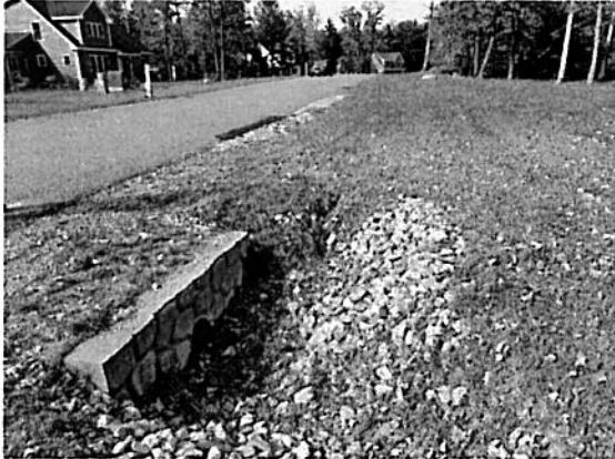
Figure 1 – Stabilize all erosion areas
