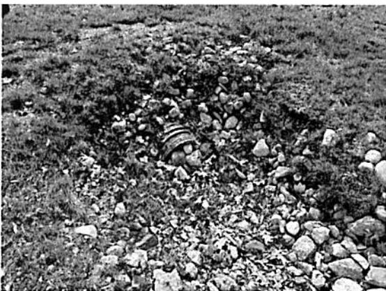
Figure 3 – Clean all outlets and drainage swales
