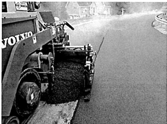
Figure 4 – Joint overlap
