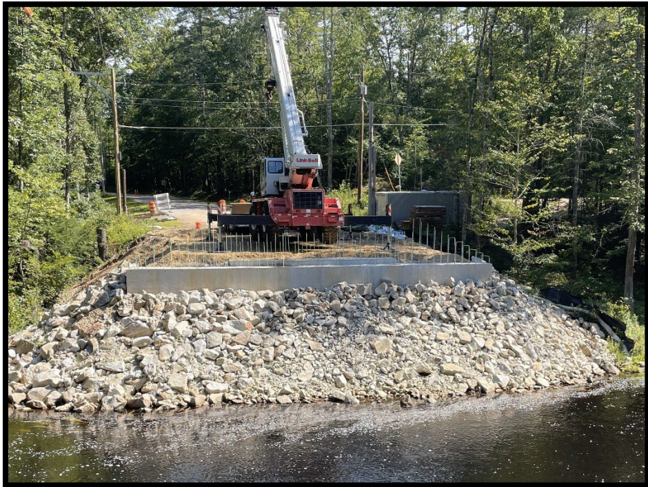
New abutment construction, August 2023
