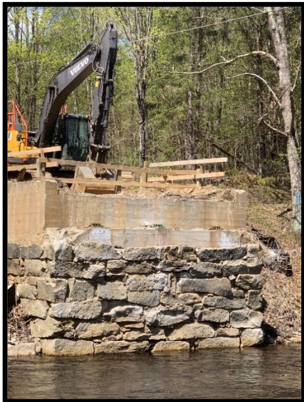
Old abutment during bridge removal
